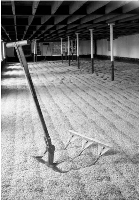
A similar malthouse still in use in Warminster. This shows the cast iron columns on the ground floor and a malt plough.
