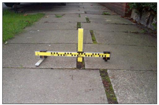
Open joint between paving stones
