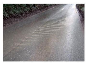
Water flowing across carriageway due to blocked highway drain
