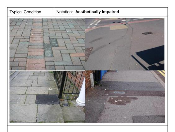
Definition: Sound footways with patching, Modular footways with sound bituminous patches, Modular footways with elements of different colour/age/material, Faded bituminous materials (especially coloured bituminous). Graffiti / Spray paint
